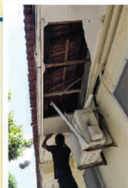
宿舍屋檐修理天花板
